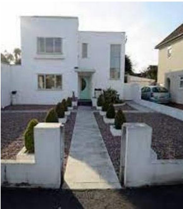
Fig.7 The All-Electric House, Bristol
