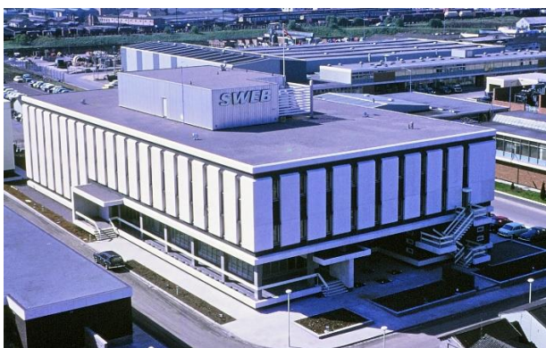
Fig.9 Feeder Road New Offices in 1970
