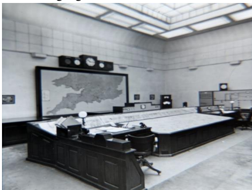
The Control room with the glass ceiling
