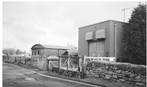
Fig.2 Old Generating Station alongside New One
