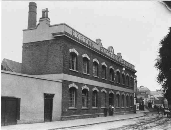
Fig.6 New North Road, Exeter Electricity Works
